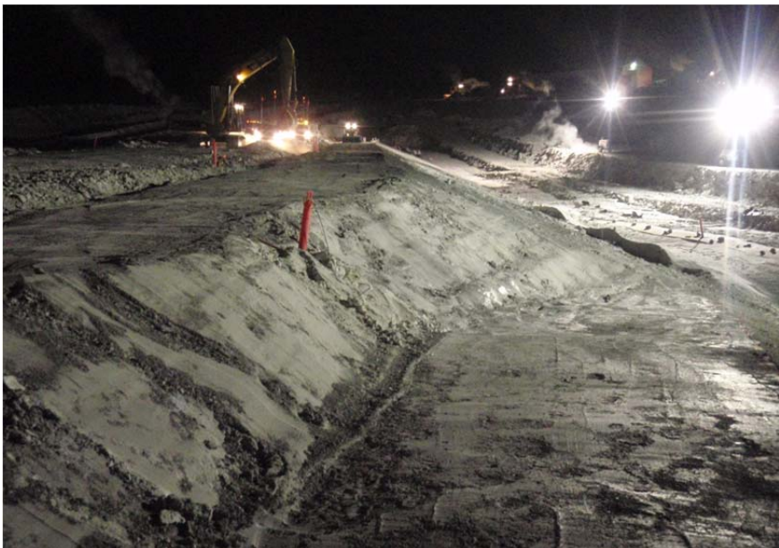
Photo 13: ~NE view of intermediate slope around 0+50 to 0+70 . at the start of dayshift. Additional cleaning of this slope was required on nightshift to remove pockets of snow, ice and loose material
