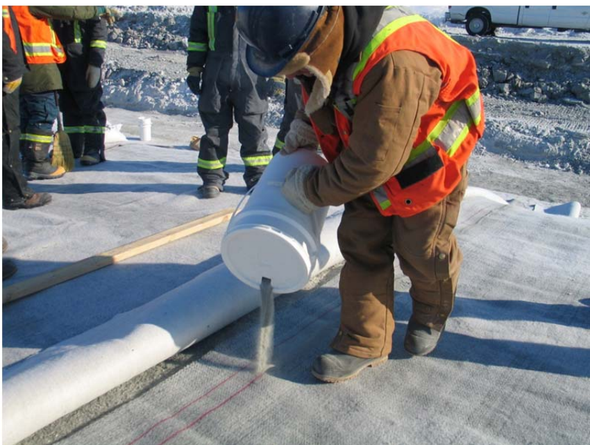
Photo 6; GCL rolled back. Placing bentonite along seam.
