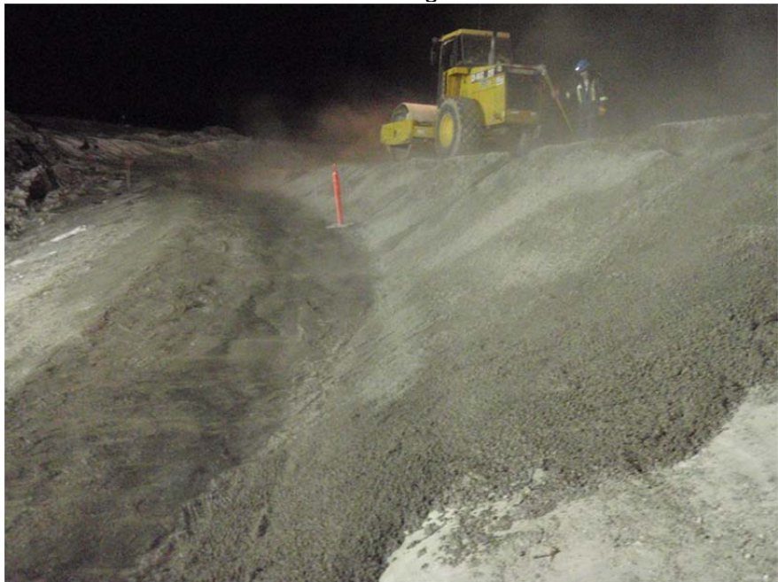
Photo 18: ~W view of SSE corner after FCM placed on side slopes to remove undulations and limit future cleaning activities.
