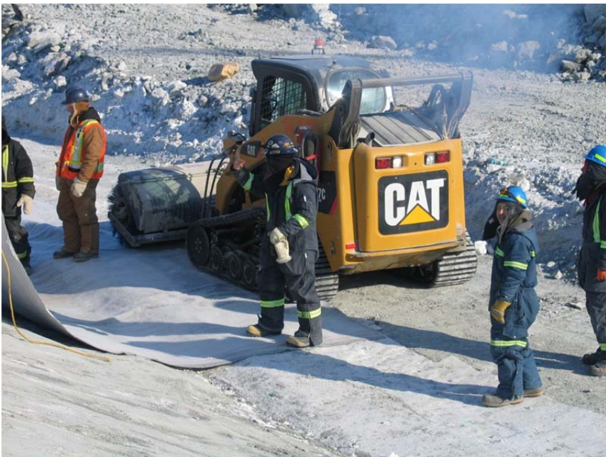
Photo 7: Skid Steer used as anchor. Note the bottom area was trimmed off after the skid steer was moved.
