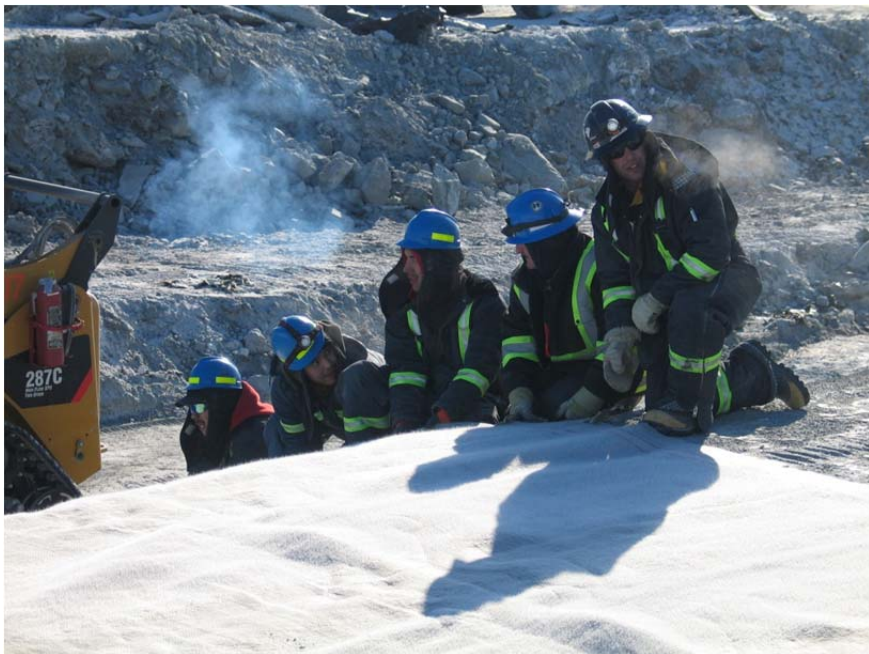
Photo 3: Workers lining up GCL panels.
