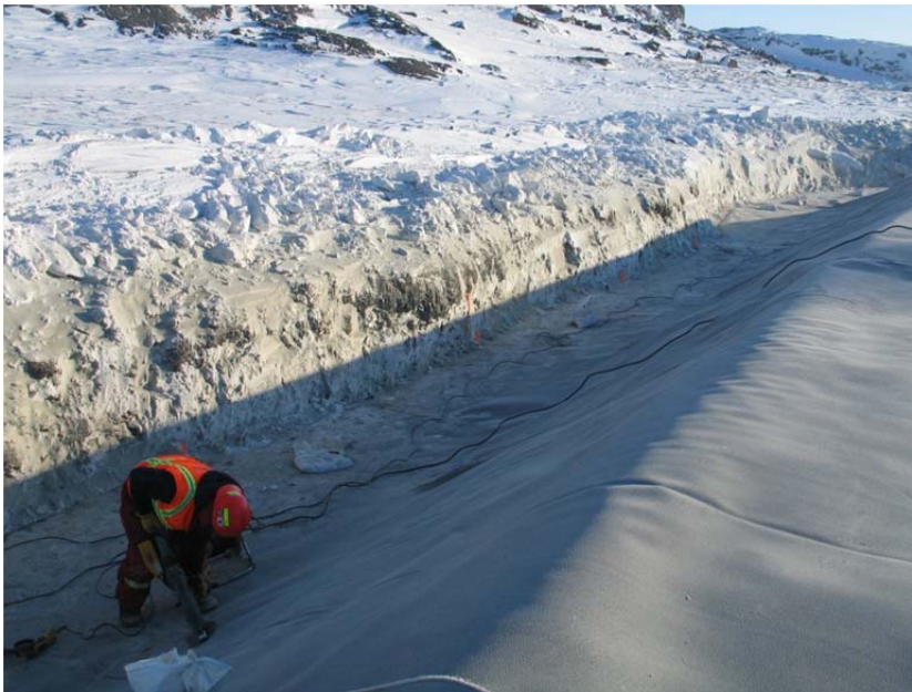
Photo 10: Geotextile Sta 3+00 to 3+45, at the DN Diversion Berm
