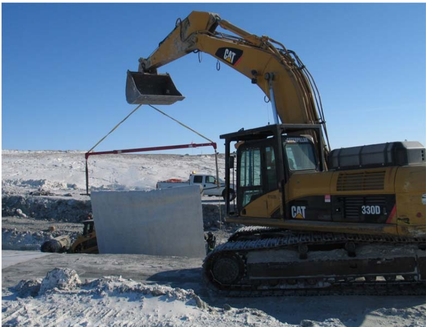
Photo 4: Cat 330 deploying GCL
