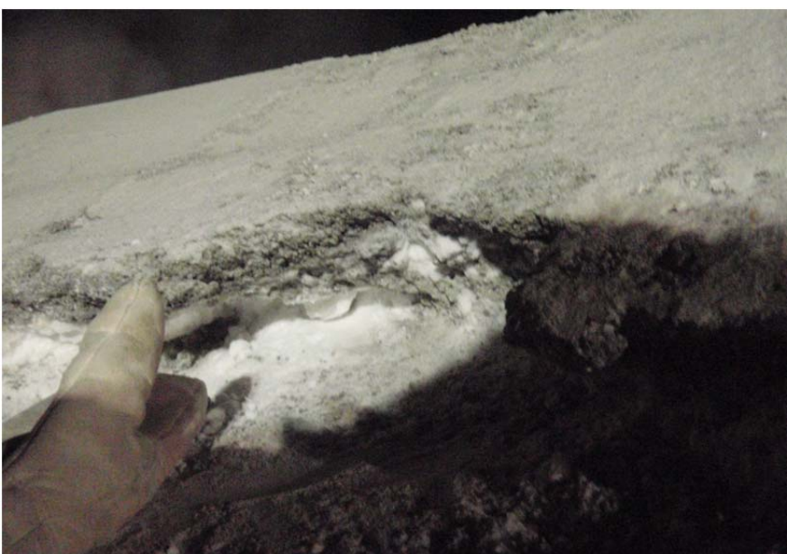
Photo 14: Example of snow pocket under FCM that fell over the side slope during the last placement. Note that this material was ripped out by the excavator
