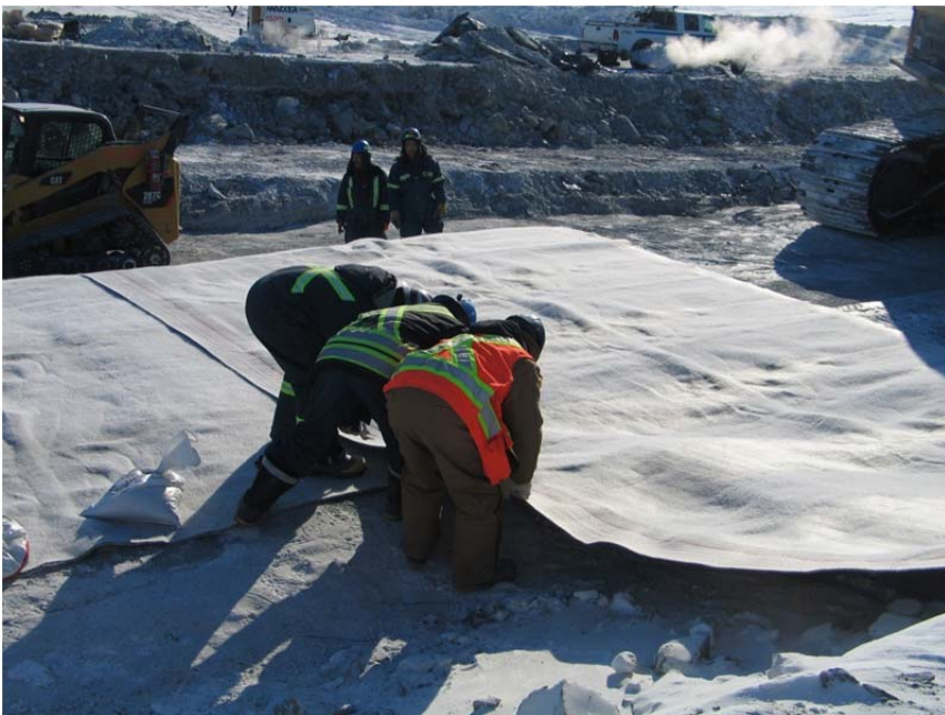
Photo 5: Workers positioning GCL after it has been rolled out.
