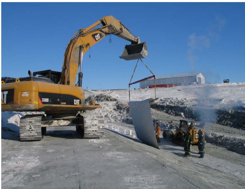
Photo 8: Labour crew and 330 spreading GCL
